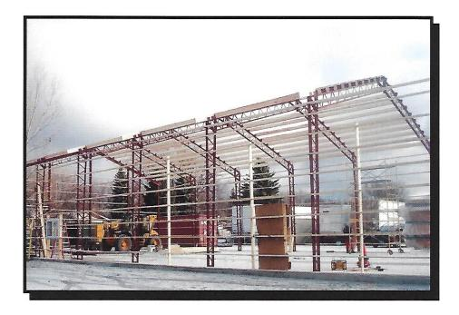
Many HBS buildings are erected by our customers. We have designed them so they go up easily using bolts and screws which are much stronger than nails.
