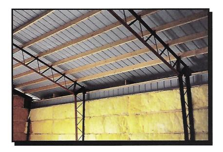
Insulating your HBS building is simple because your outside sheet steel and inside columns/ trusses never touch. Purlins and girts are 24 inches on center with 6 inch wall spacing & 8 inch ceiling spacing. Installing insulation, even years later, is simple.
